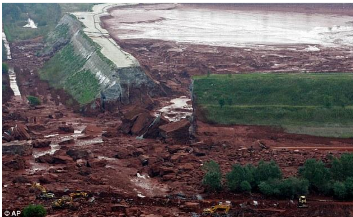
Figure 6 Collapse of Red Mud Impoundment Facility in Hungary. Source: Mines and Communities website
