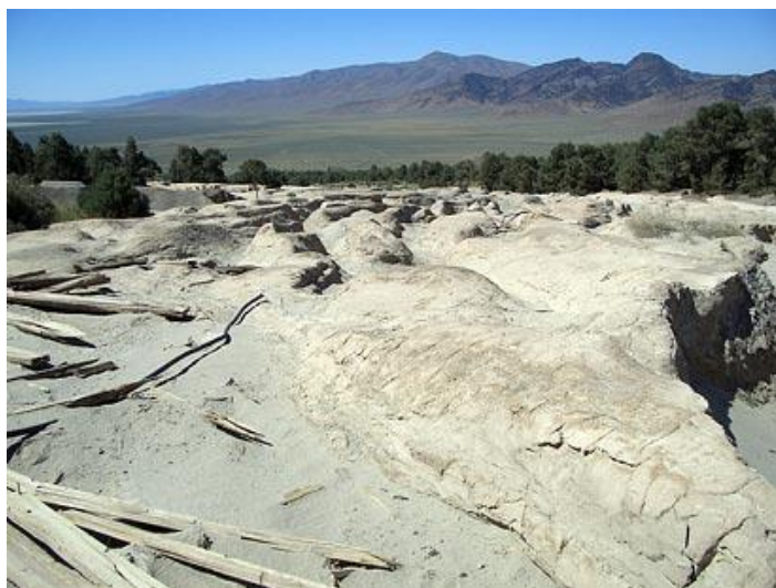
Figure 9 Riverine disposal in abandoned gold mine in Nevada, USA. Copyright Jon Engels
